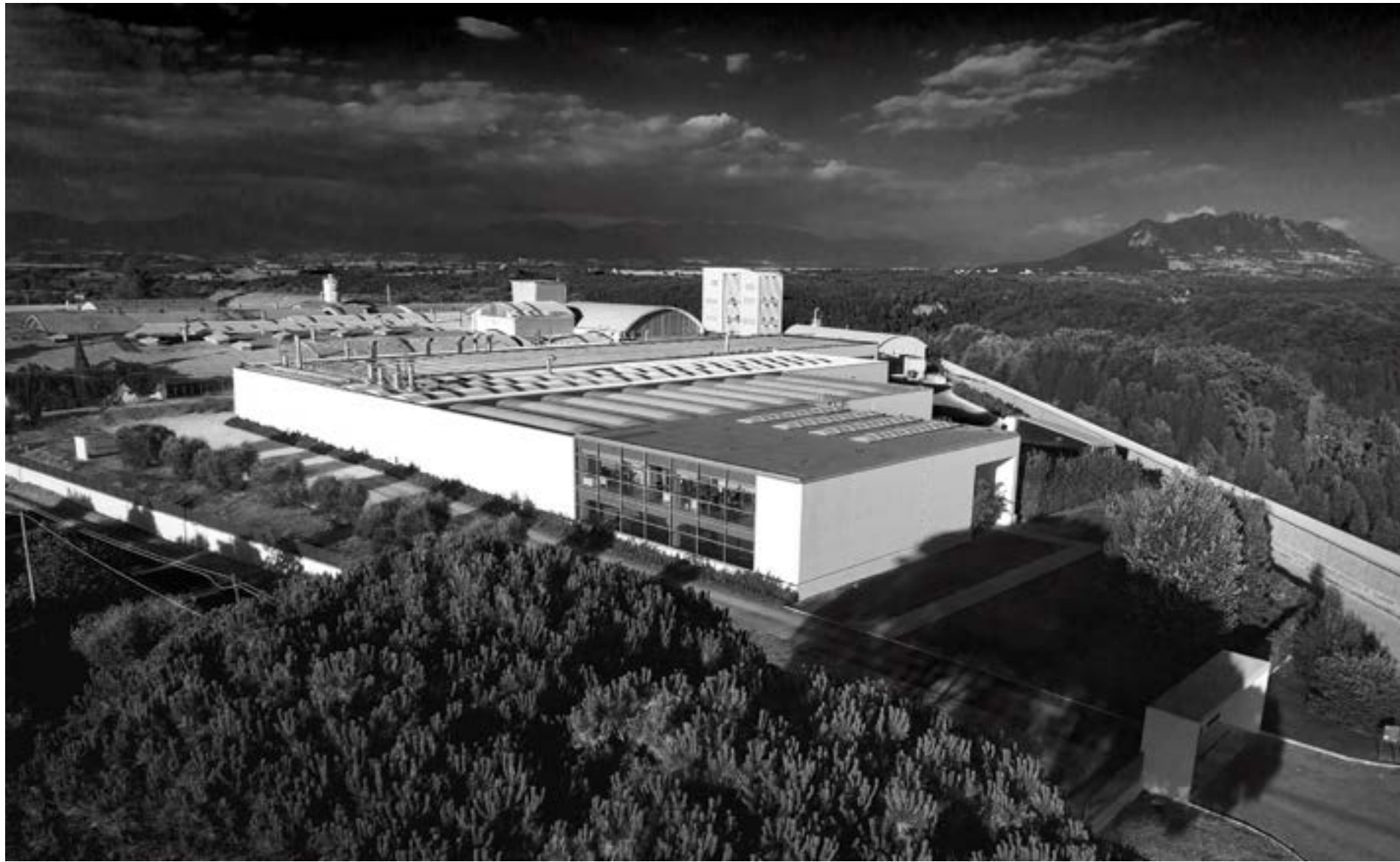
Headquarters and Factory, Castel Sant'Elia – Italy
